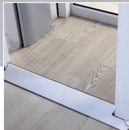
Sloped threshold and attractive non-skid flooring
